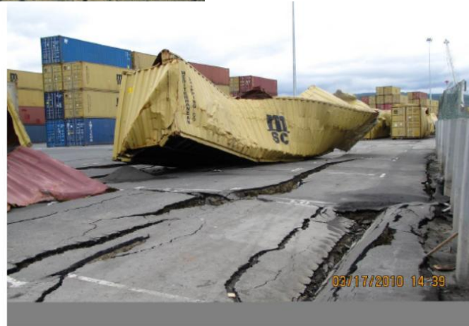
Figure 8.3. Photograph of lateral spread displacements at the Port of Coronel. The wrecked container was part of a stack and was ejected in front of the sheet pile wall, passing through the barbwire fence above the wall. It was subsequently recovered from the beach and brought back to the dock using a crane (S37.028680°, W73.150054°, 1440 hrs, 03/17/2010).
